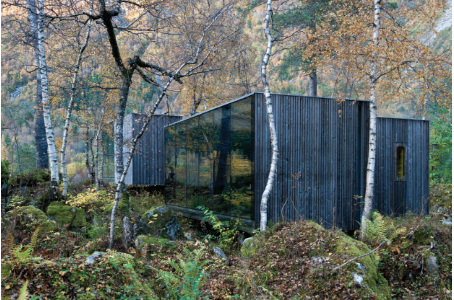
Juvel's cubes are built on stilts to highlight their temporary nature
